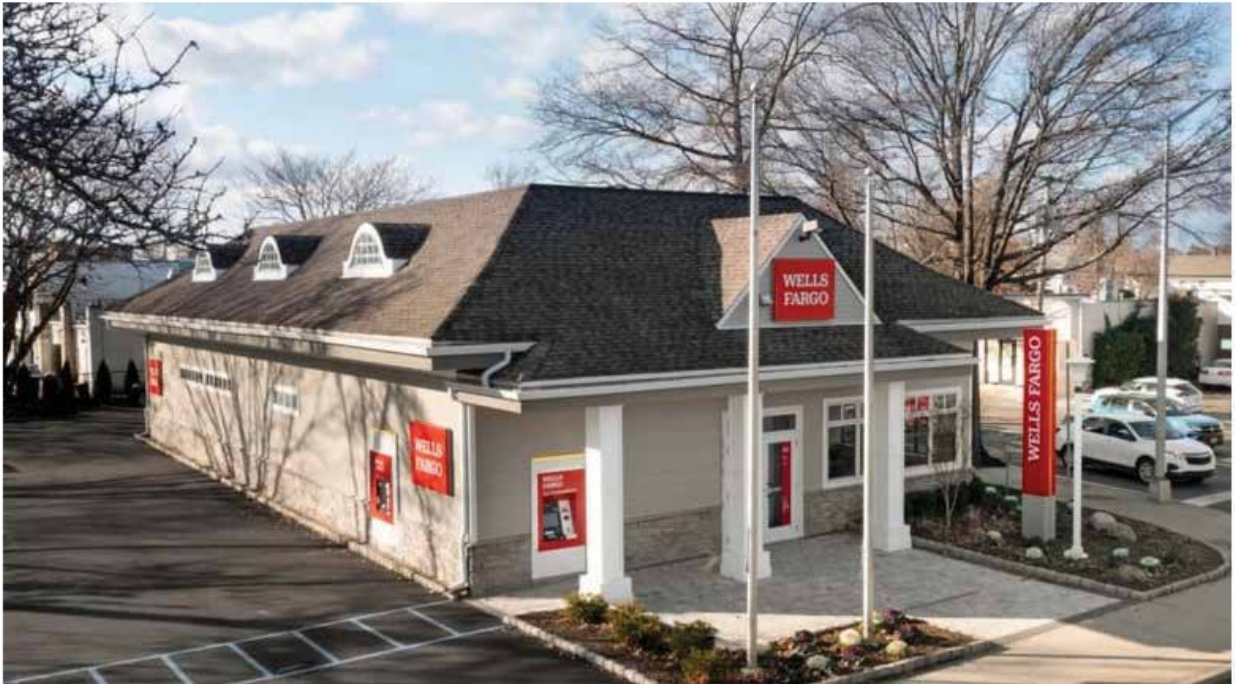
The new Wells Fargo branch in Port Washington. (Photo: Wells Fargo)
